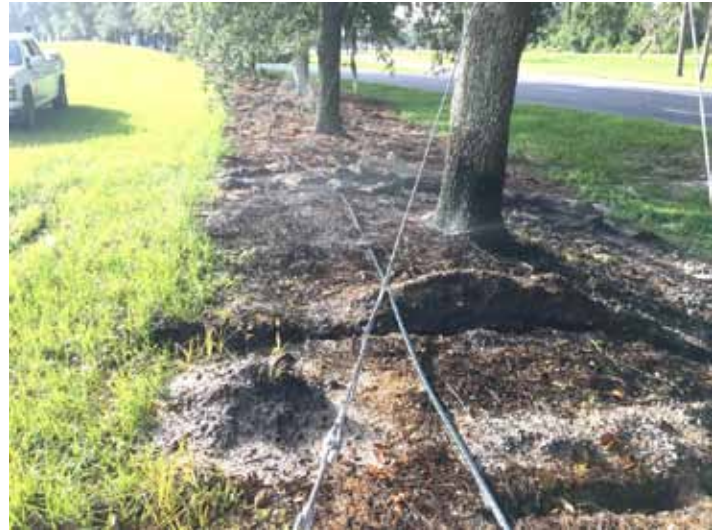
Picture #3. Root pruning in advance minimizes tree stress. Digging a double set of trenches around the tree makes it easier to remove the cut roots later on. Note guying cables and supplemental irrigation in picture.
