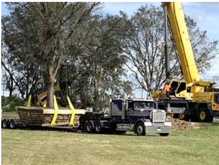
Picture #5. Most of the trees needed cranes and lowboy trailers for loading and transporting.
