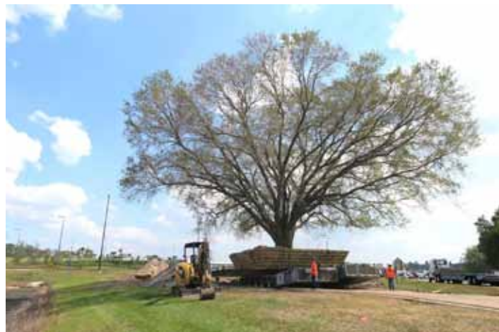
Picture #6. Sixty inch trunk diameter Live Oak transported by two "Smart" trailers in tandem. This picture shows the trailers poised to drive the tree down the ramp into it's final planting location.
