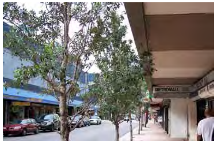
Figure 1.- Bad design, large trees too close to the building. Photo courtesy of H. Mayer.
