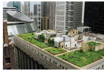
Figure 4.- Green Roof of Chicago City Hall, courtesy of Chicago2
